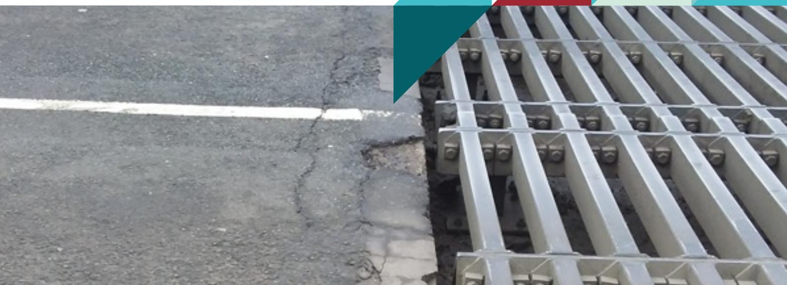
When nosing concrete breaks out below the level of the grid, it creates an impact point for traffic on the face of the grid steels. This can compromise the grid anchor points – an expensive fix. Remedial action is essential.
