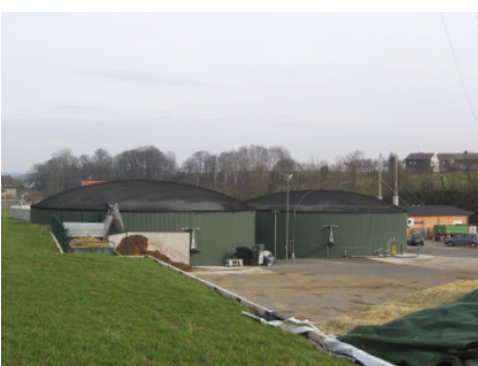
Biogas plant in Brakel, North-Rhine-Westphalia
