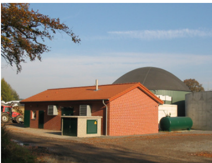
Biogas plant in Velen, North-Rhine-Westphalia
