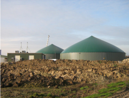
Biogas plant in Gusow, Brandenburg
